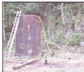
The same well after installing an Airwell pump.
